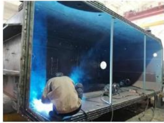
Main transformer Oil tank production
