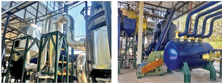
Gasification technology is the use of biomass fuel to burn in a specially designed furnace which is called as “Gasifier stove”, it will control the amount of air entering the furnace in lesser volume than usual to force the situation which is called “Incomplete combustion”. Such condition will cause the heat inside the stove approximately 1100 degrees Celsius and there are five types of gas occurred:
